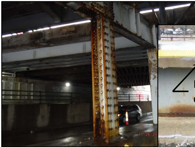
Center Steel Pier
