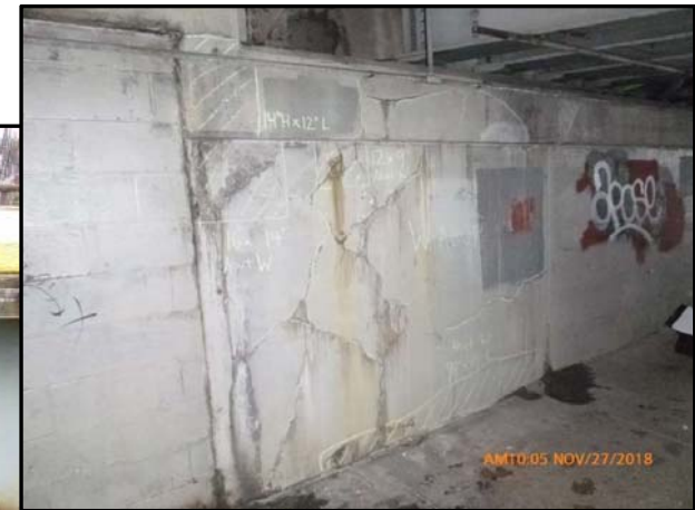
Concrete Foundation @ Ends
