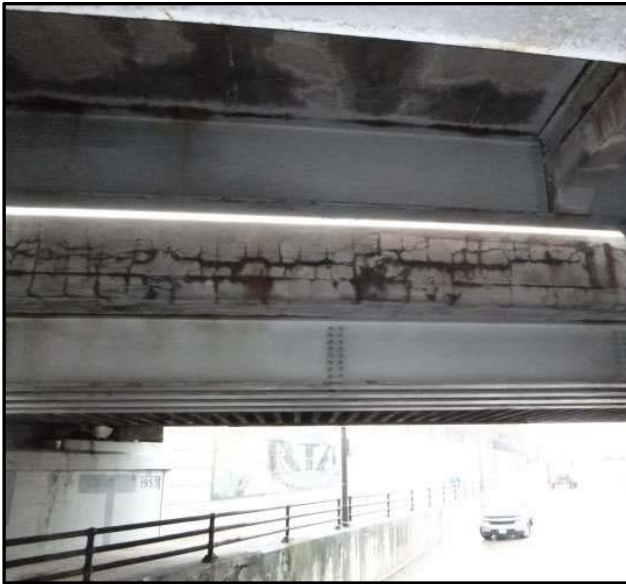
Concrete Deck on Steel Beams
