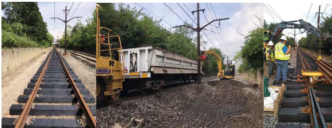
Figure 62: Light Rail Ongoing Track Rehab
