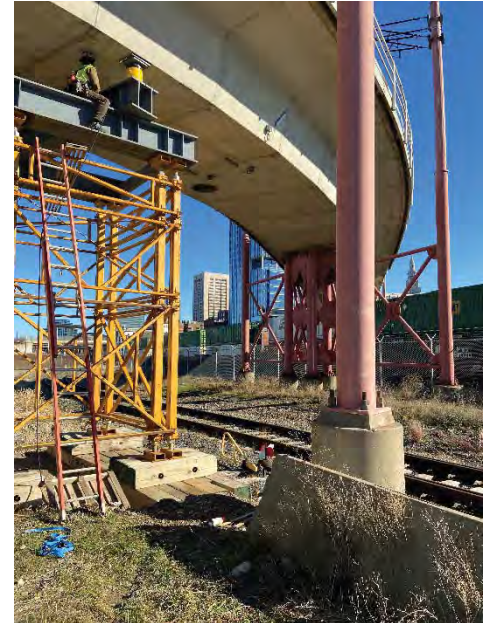
Figure 45: Jacking Process on the Waterfront Line Bridge
